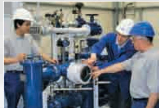
Commissioning and training by Lechler staff
