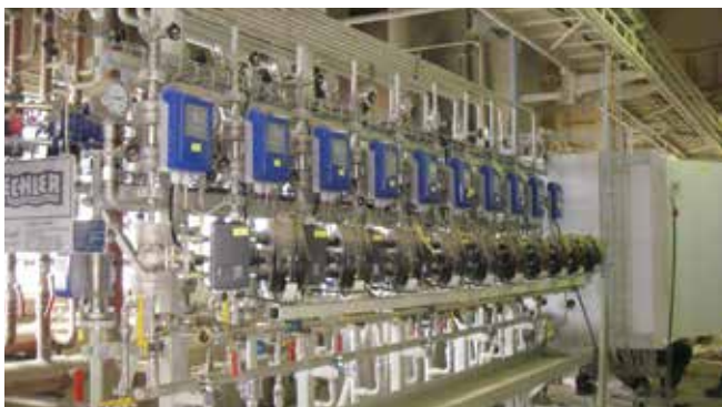
Controlled section of a heSNCR
